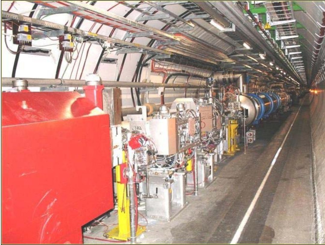
Figure 3: Beam instrumentation, collimators and other equipment presently installed in between the TAN (red object on the left) and the D2 separation dipole (blue cryostat on the right) in the ATLAS matching section.
