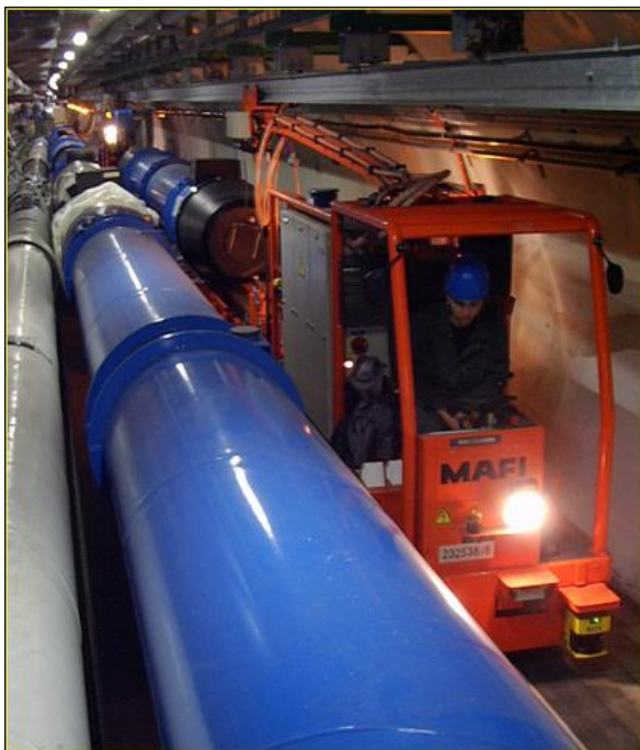
Figure 3: Transport of magnets in the LHC tunnel.
