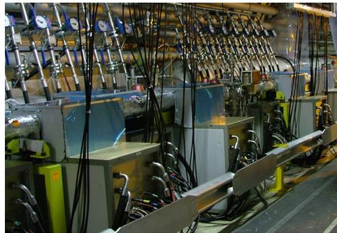
Figure 2: Kickers and amplifiers in the LHC tunnel.
