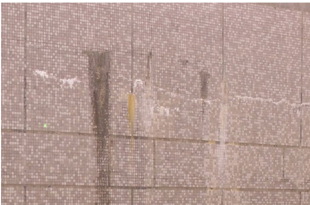
Figure 6. The close-range horizontal photography by UAV's camera
