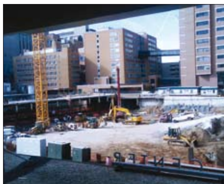
The construction site of the Genome Sequencing Center's new computer centre in St. Louis. Courtesy of Andras Horvath.
