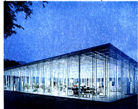
Figure 28: The new workshop at KAIT (Source: Architectural Record)
