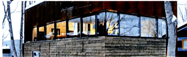
Figure 19: Hokkaido Tracks' 2009 Hirafu House
