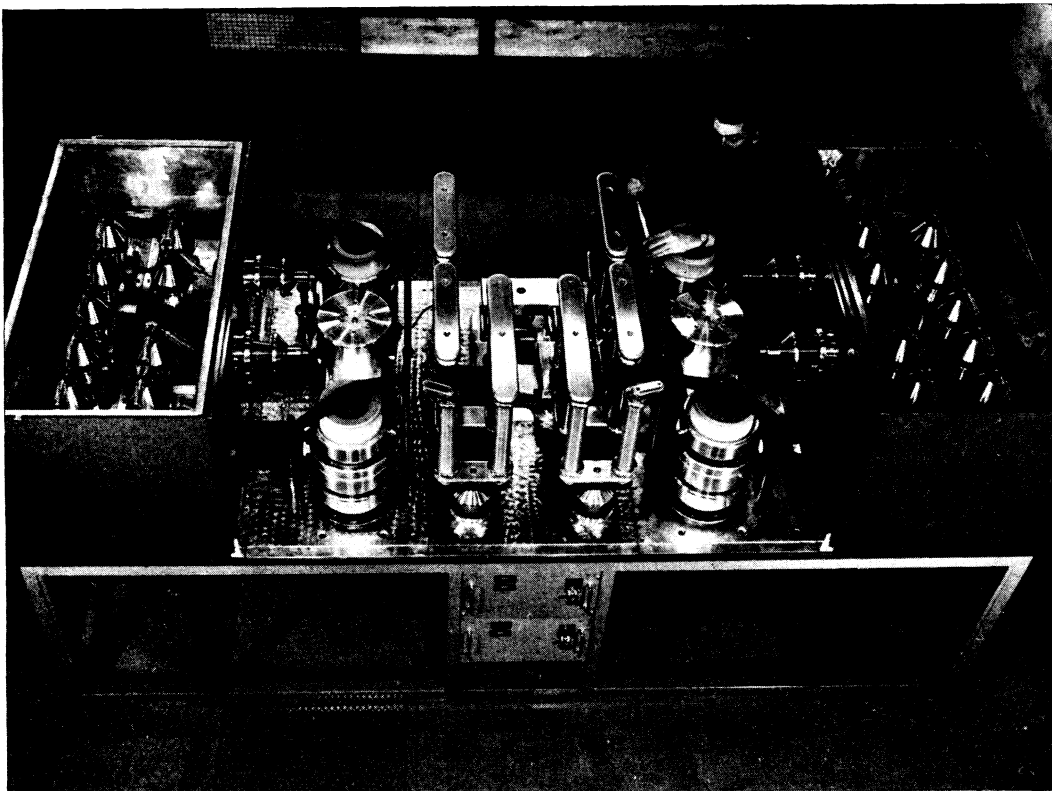
FIG. 3. Pulser of the present CERN PS kicker. Two storage networks can be seen at either end. Switching spark gaps and high voltage components are inboard of the networks. (Credit: CERN PHOTO)
