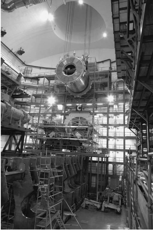
Fig. 1. Descent of the Barrel Cryostat with solenoid and calorimeter into the underground cavern.
