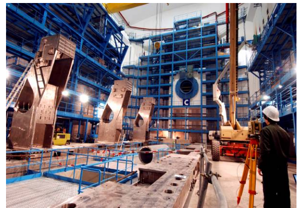
Fig. 21: Adjustment of barrel toroid feet after the precise adjustment of the bed-plate
