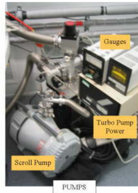
Figure 3: Vacuum pump system
