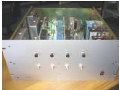
FIGURE 20: Signal processing electronics located in the hall
