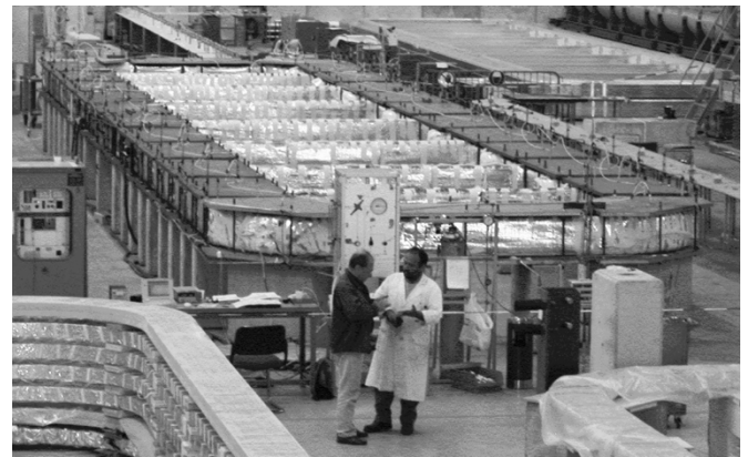
Fig. 4. A completely assembled cold mass during the curing under pre-stress operation.
