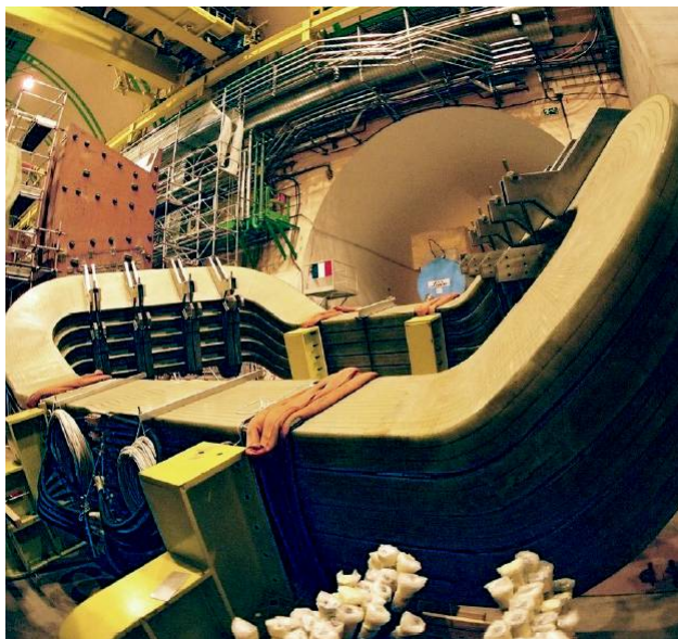
Figure 1.11: The installation of the magnet in the LHCb cavern.
