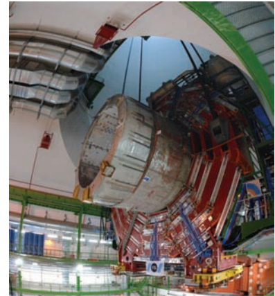
Figure 2. Lowering of central wheel with magnet coil.
