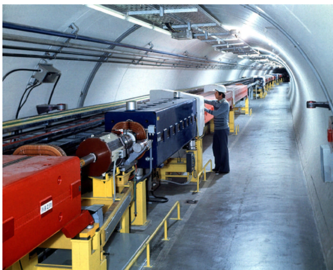
Fig. 11: View of the SPS tunnel with dipole magnets (red) and quadrupoles (blue)
