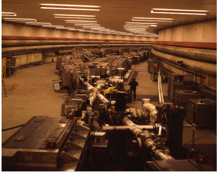
Fig. 7: View of the ISR at intersection point 5
