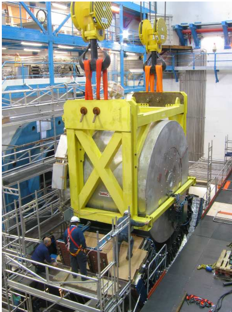
Figure 18. One of the two end-cap cryostats being lowered into the ATLAS experimental cavern. The entrance to the LHC tunnel can be seen on the left, partly hidden by the cryostat.
