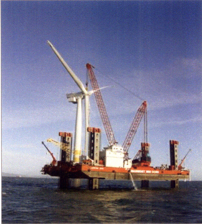
Figure 3 Offshore Wind Turbine Installation
