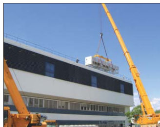
Clockwise from top left: Removing the old cooling towers... three new chillers waiting to be installed... going up... and in place on top of B513.
