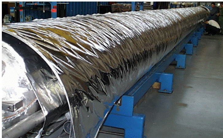
Figure 10 Prefabricated MLI blankets being installed around an accelerator superconducting magnet
