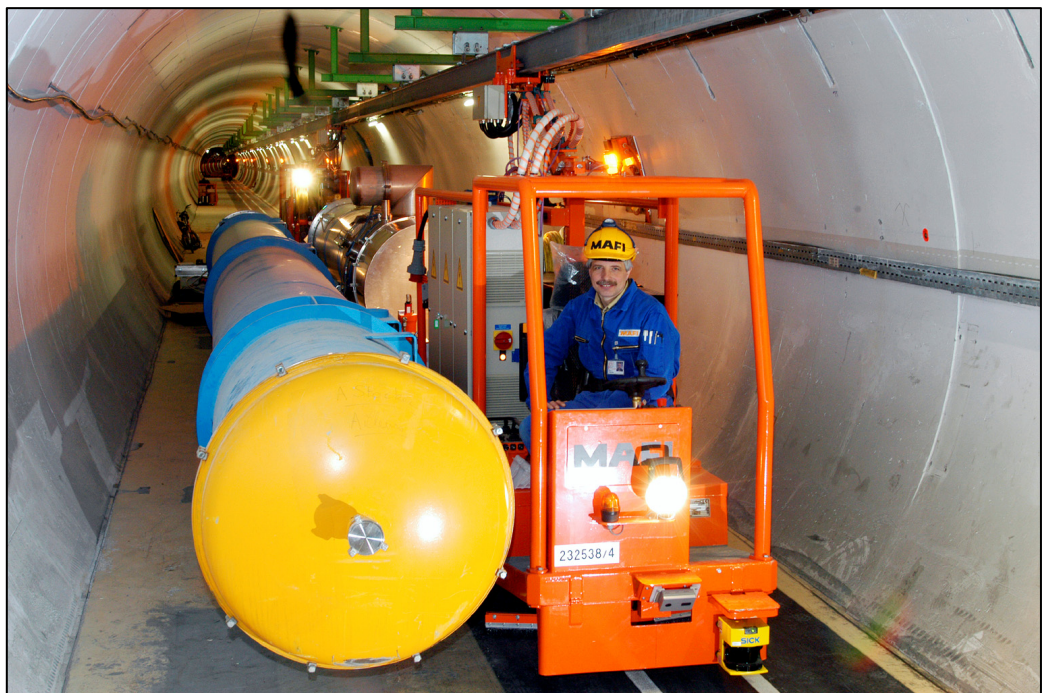
Dipole magnet transport in the LHC tunnel.
