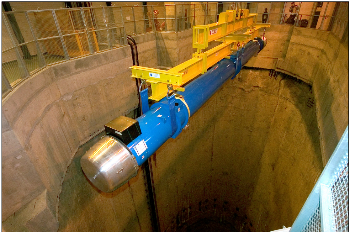
The first LHC dipole magnet lowered into the tunnel.
