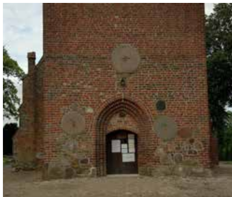
Figure 6: Three medieval millstones embedded into a wall of the Gothic church in Osiek Koszaliński (photograph by D. Brykała, 2019).
