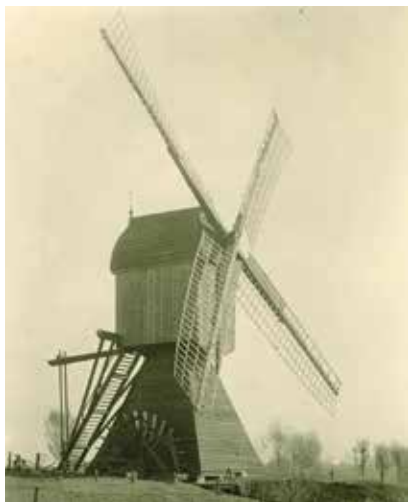
Figure 3: A draining windmill in the area of Żuławy. Picture from the early twentieth century (from the resources of Marienburg Archiv, Hamburg)
