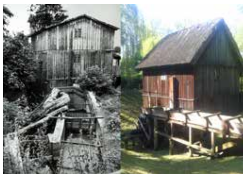
Figure 4: Watermill from Strzygi with: a turbine (left – in situ in 1960s) and a overshot waterwheel (right – ex situ in 2014). Currently in the Ethnographic Museum in Toruń (photograph by Archive MET, sign. I-1306-90; K. Koczyński 2014).
