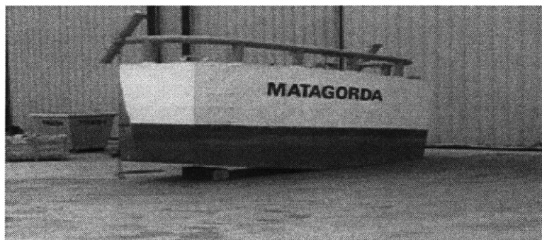
Figure 23: The 5' stern section of the Matagorda at the shipyards in Lockport, LA soon after it was cut as part of the upgrade.
