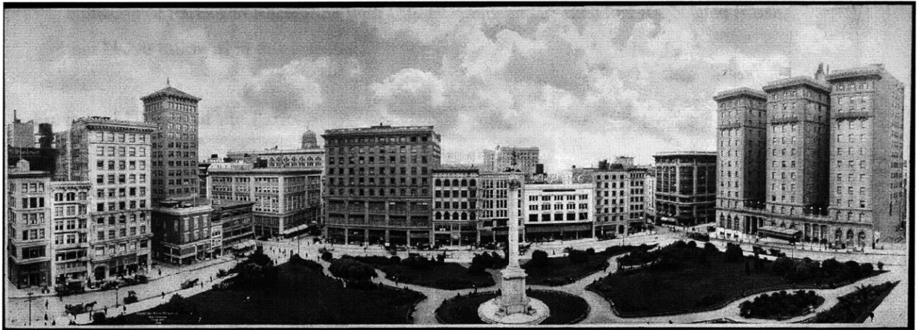
6. Union Square Panorama, c. 1870, looking north from 14 th Street
