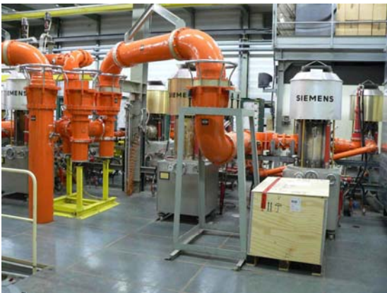
Fig. 7: Amplifier of 135 kW (right, tube below the ‘hat’) coaxial RF lines and hybrids (SPS)
