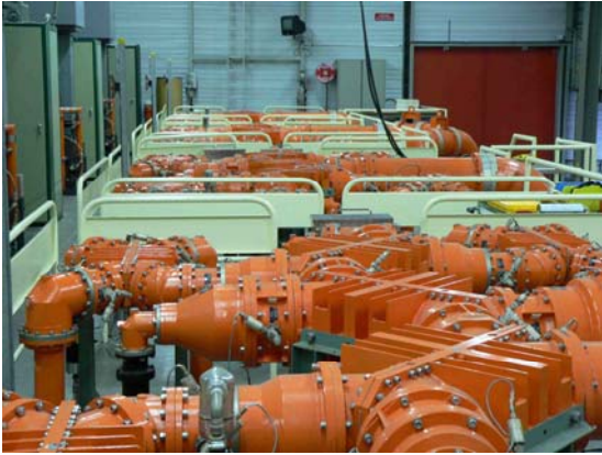
Fig. 6: RF hybrids ‘joining’ the RF power flux (SPS)
