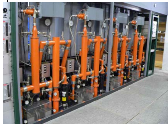
Fig. 5: Racks with 4x2 gridded tubes of 35 kW (nominal) at 200 MHz (SPS)
