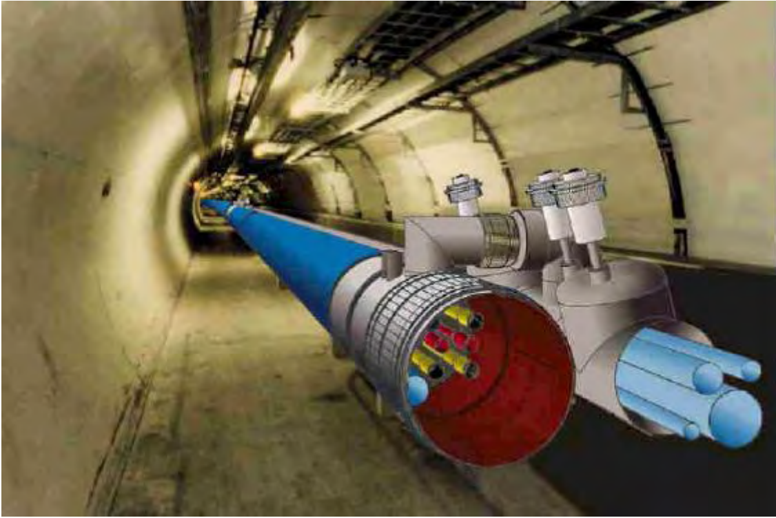
Figure 2.3: The magnet and the QRL in the tunnel, visualized open-ended
