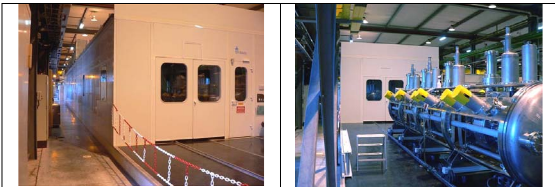
Figure 4: Picture of cleanroom for LEP- and LHC-module assembly. It is divided in two parts of equal size, each 15 m long and 4 m wide, separated by a large double door. The dust-filtered air is blown from the ceiling towards the floor. The entry part is in class 1000, and the working part is in class 1÷10, exceptional for an installation of this size. An object enters the front part, letting the dust settle, and is only then transferred into the main working part. Right of the main doors, the personnel entry door to a small space for the operators to change into special garments, with another exit door into the class 1000 zone. The 'front court' allows modules to be mechanically assembled or disassembled (critical volumes remaining closed, only opened inside) and set onto rails; these lead along the whole clean-room for easy transport.
