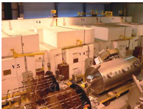
Figure 3: Vertical test cryostat area. Visible are only the concrete 'hats' for radiation protection. These can be rolled away on rails, uncovering below a test cryostat sunk into the ground; two with sufficient depth to contain a LEP 352 MHz cavity of 2.4 m length and the (heat) radiation shields above it, and one of lesser depth used for single cell cavity tests. The 300 W solid-state RF power amplifiers with their circulator and load are housed behind the concrete wall (for low power cavity/module tests)
