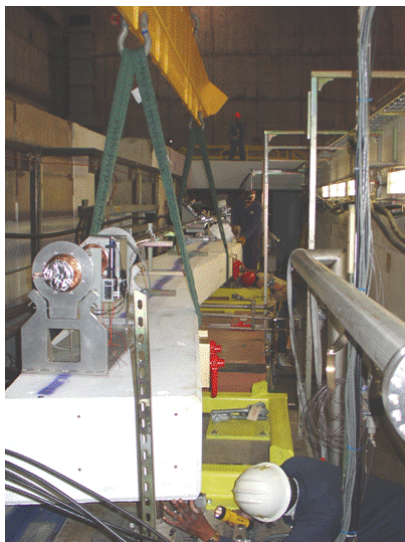
Figure 2: Installing the girder supporting the BPM3-5 triplet.
