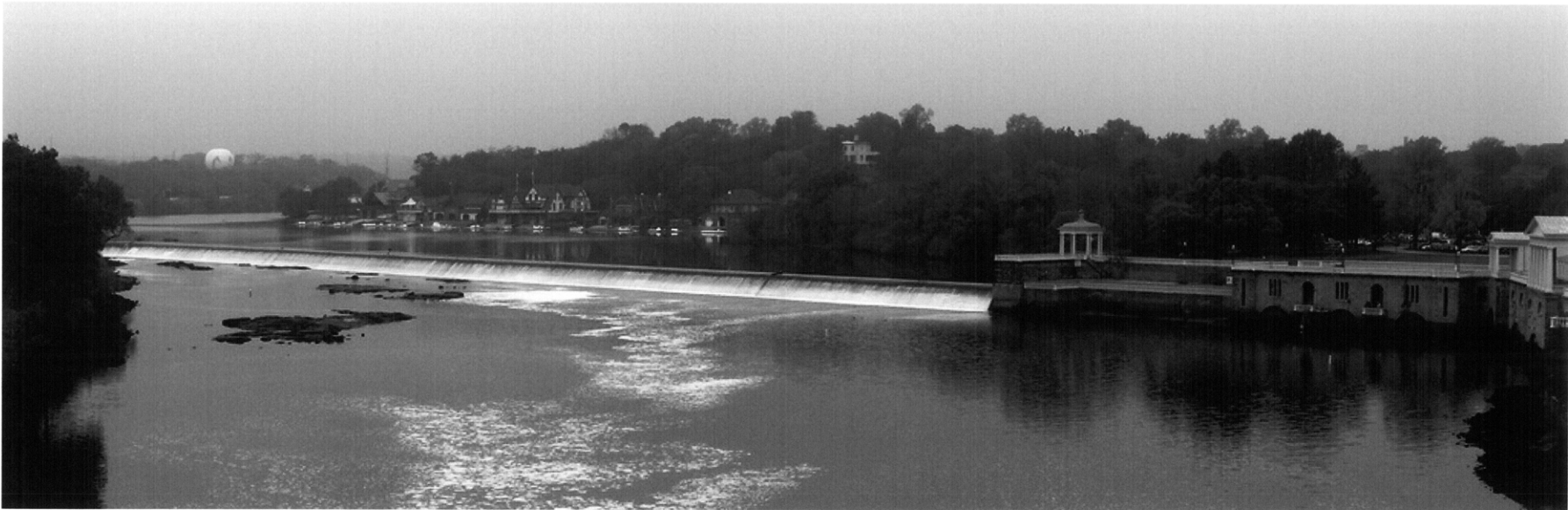
Fairmount Waterworks and dam looking west across the Schuylkill River
