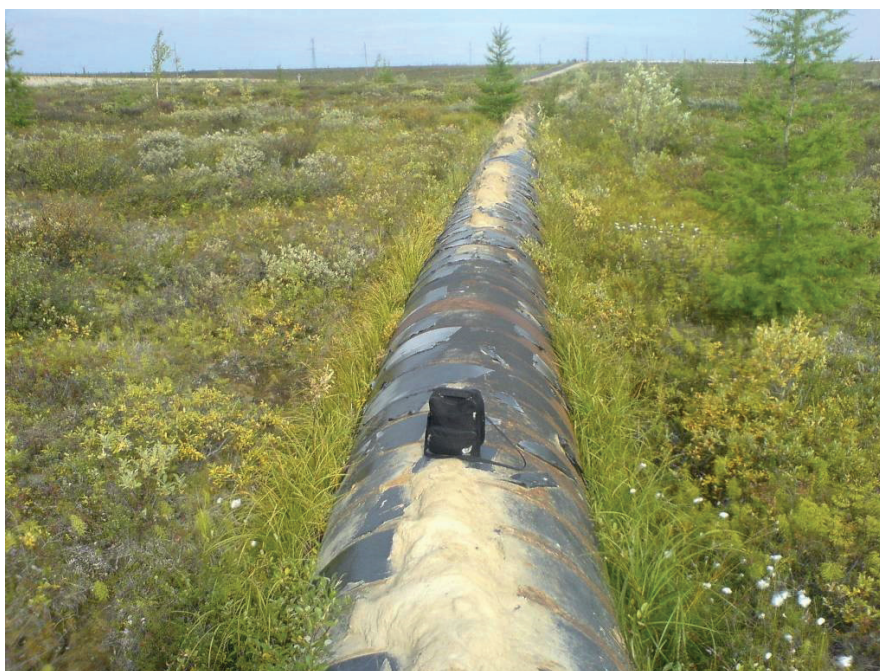
Fig. 2. The pipeline section without deboning
