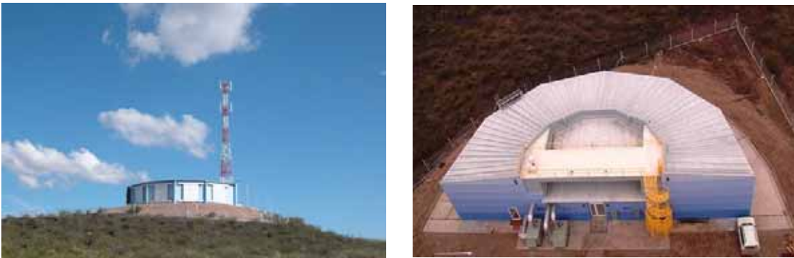
Figure 4. Two views of one of the fluorescence telescope enclosures. The view on the left includes the enclosure with shutters and the communications tower in the background. The view on the right is taken from the tower and shows the 6 – 30° telescope bays.
