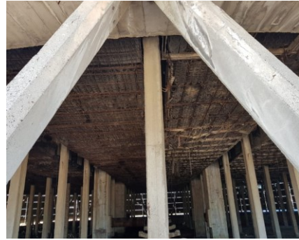
Fig. 4. Cooling tower at the base side.
