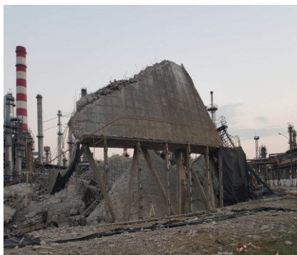
Fig. 10. Tower after demolition - back view.
