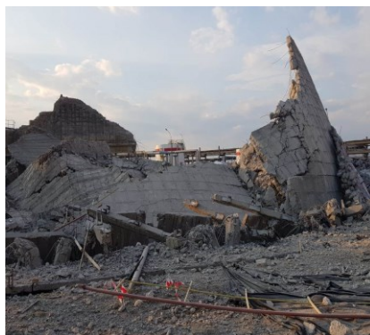
Fig. 11. Tower after demolition - lateral view.
