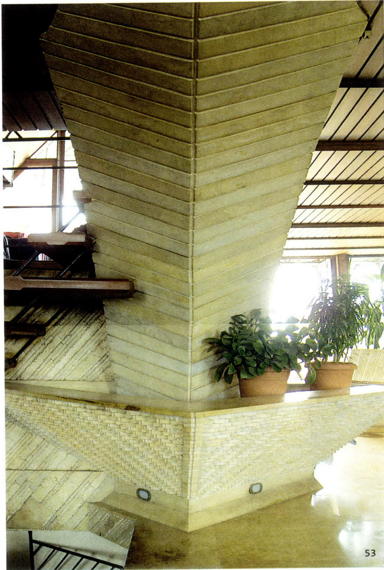
Left: The triangular arch tried by Nari Gandhi at the Azmi Penthouse. This was later tried again on a larger scale at Tungarli.
