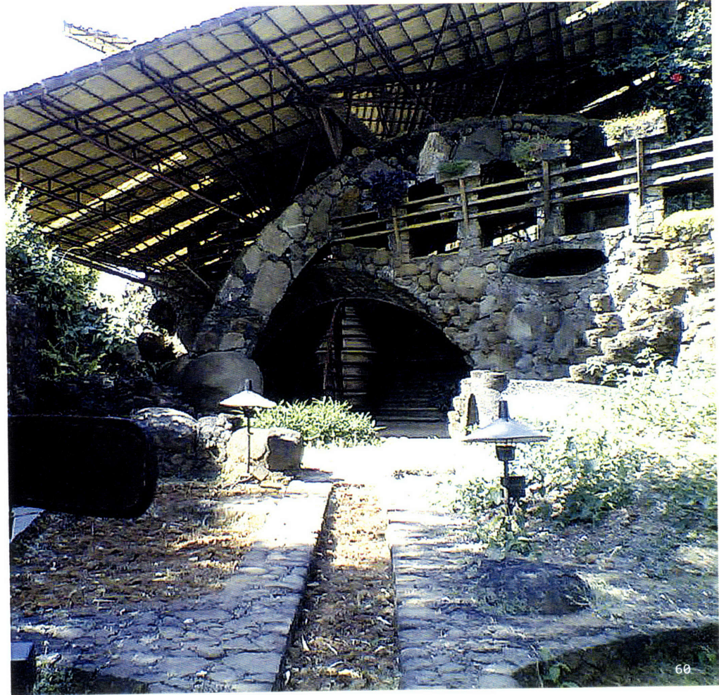
Tejani's Tungarli bungalow follows an arcuate structural parti with stones of all sizes rising from the ground and making the house. Details are done in chipped-stone with glass and smoother rocks
