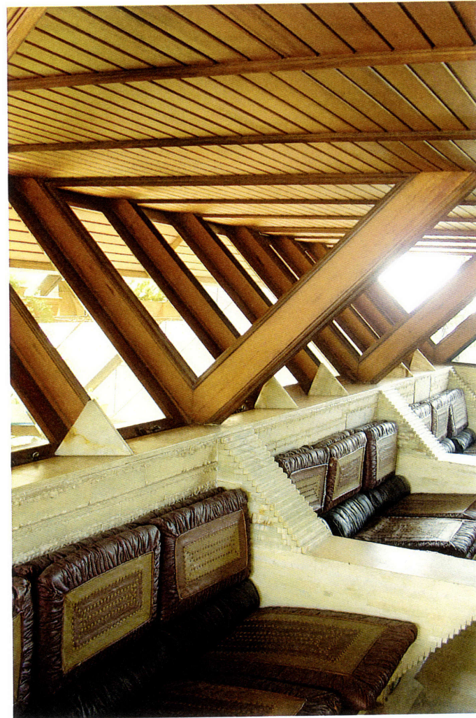
Left: The triangular arch tried by Nari Gandhi at the Azmi Penthouse. This was later tried again on a larger scale at Tungarli.
