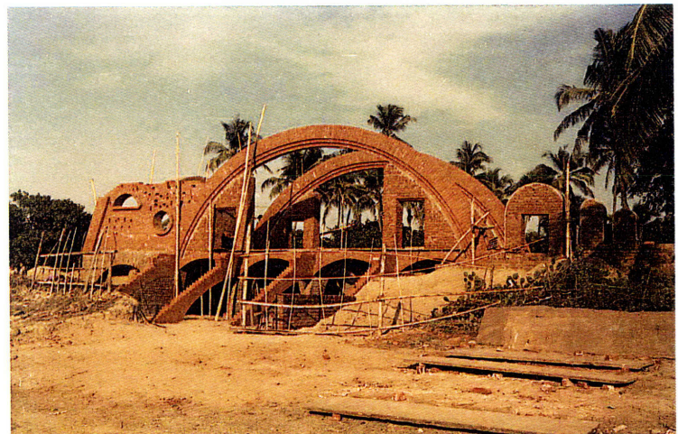
Below: left and right: Photos show intermediate stages of construction. The main arch and buttress were constructed first - and piled sand is used as landfill during construction
