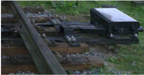
Fig. 3. External view of the SP-6m turnout
