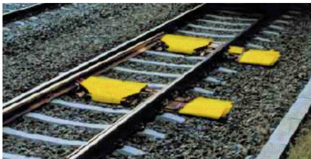
Fig. 1. General view of the EBI Switch 2000 turnout
