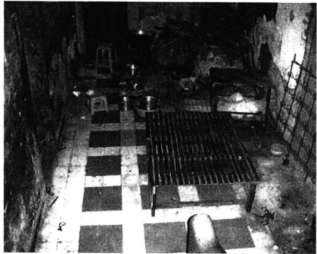
Squatting in a corridor inside a building
