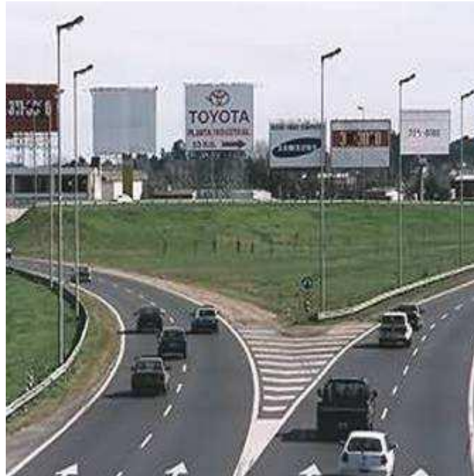
FIG. 8 Areal View Of The Northern Highway
