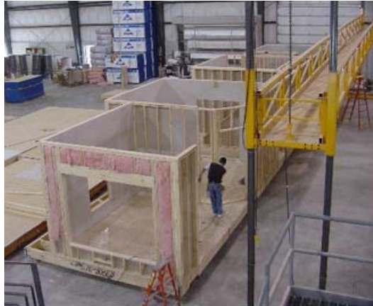
Figure 9: Prefabrication at Warehouse
