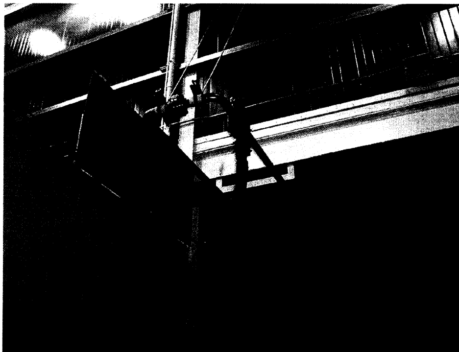
Fig. 27 20 kA cables and water cooled resistor to improve the stability of the voltage power supply.
