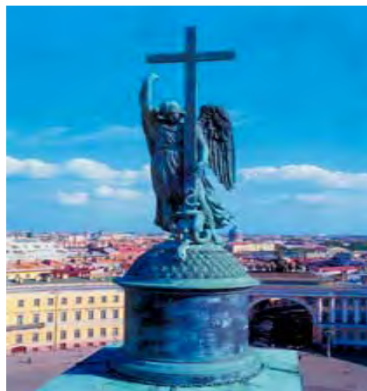
Fig. 2. Bronze angel from the top of the Alexander's column covered with greenish stain, Sankt-Peterburg.
