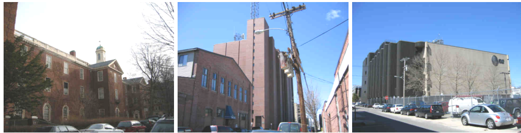
Figure 10: Cambridge TelData Buildings
