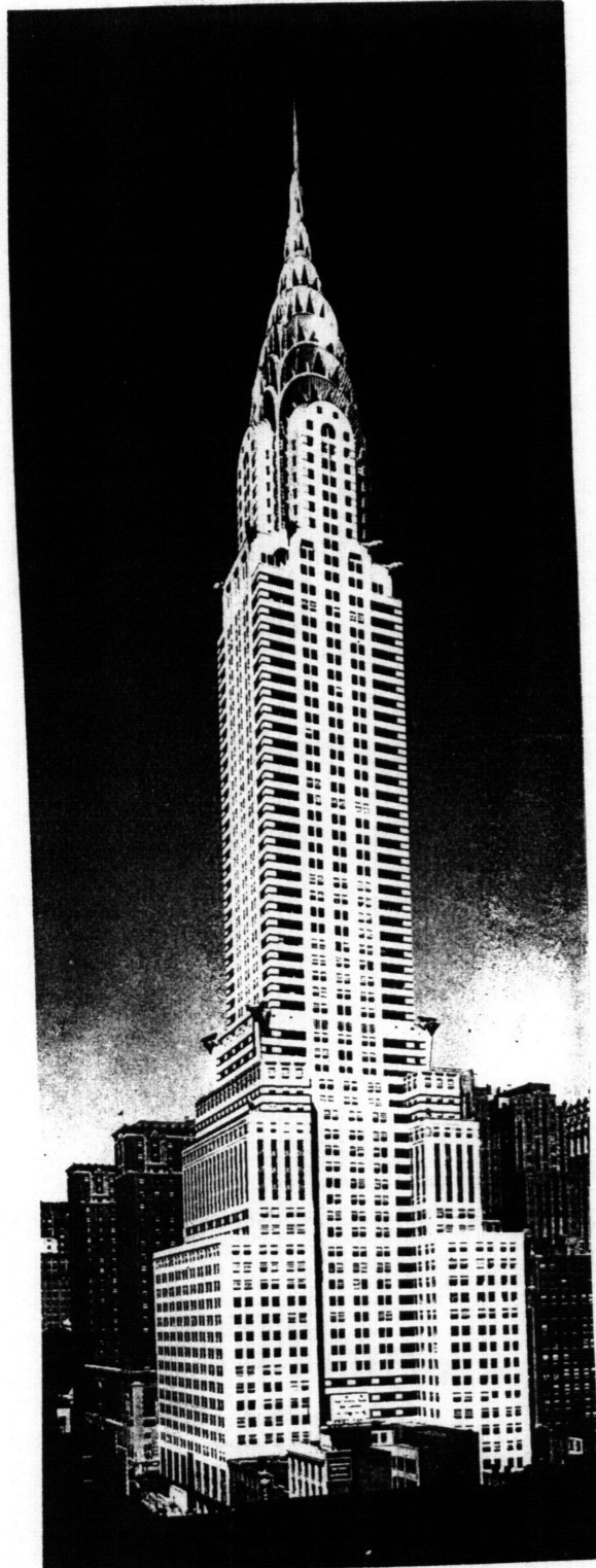
Figure 1.4 -- The Chrysler Building (1928-1930) Lexington Avenue and 42nd Street
