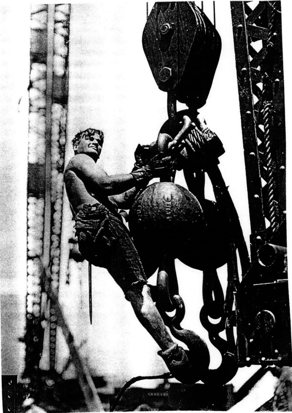
Figure 2.4 -- Construction of the Empire State Building (Photograph by Lewis Hine)
