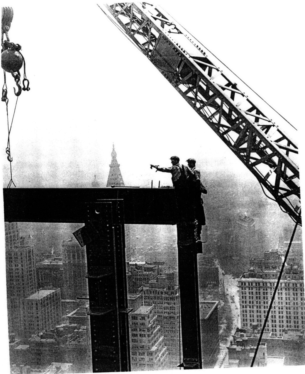
Figure 2.2 -- Construction of the Empire State Building (Photograph by Lewis Hine)
