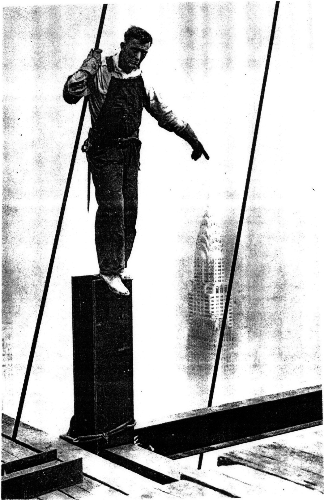
Figure 2.3 -- Construction of the Empire State Building (Photograph by Lewis Hine)
