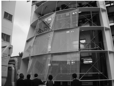
Figure 2.11b: Full Scale mock-up to evaluate translucencies of glass panels, Entry Structure (2003)
