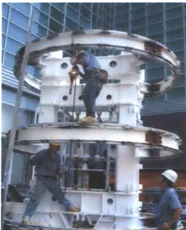
Figure 33: Workers Installing Pinnacle TMDs; Picture courtesy of Motioneering Inc.
