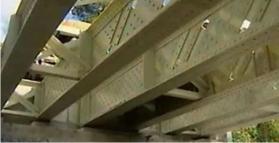
Fig. 3. Fragment of a road bridge superstructure made of composite polymer material.
