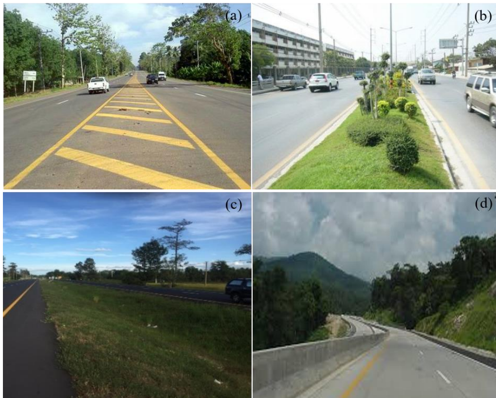
Figure 1 Road median type (a) Flush median; (b) Raised median; (c) Depressed median; (d) Barrier [2]
