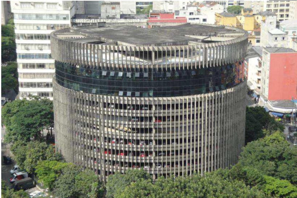
Figure 8. Air view of the Alfredo Issa multistory parking garage in the 2000s before preservation issues became more and more serious. Please notice the change in the volume with the inclusion of two other floors, a new top design that preserved the idea first conceived plus a helipad, which was soon deactivated. Private Collection.
