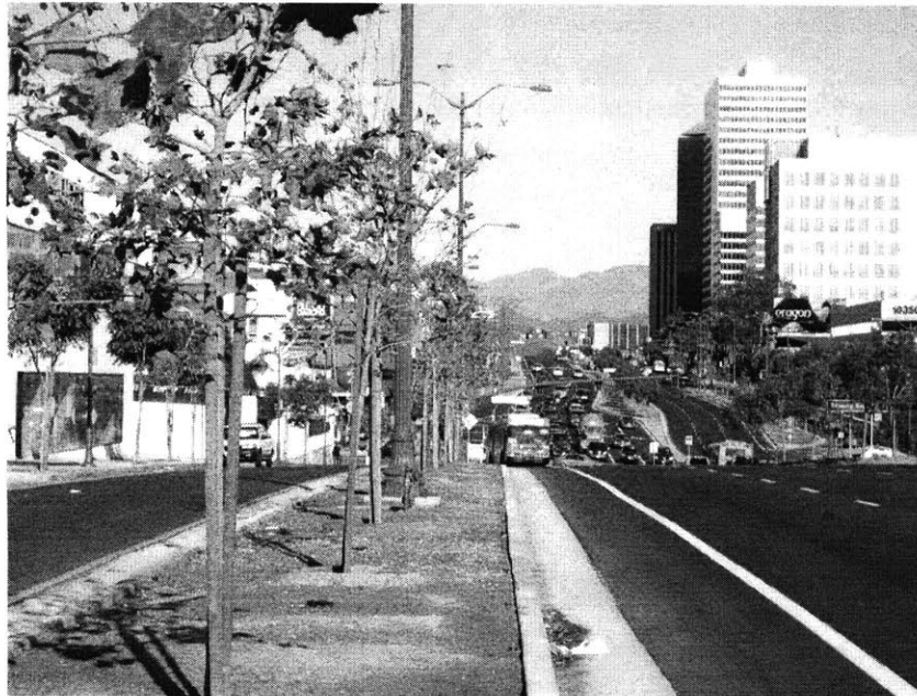
Figure 6-26: Some of the more unconventional designs on Santa Monica Boulevard: narrow medians with trees, side access lanes for local traffic, six-foot bicycle lanes (looking east); Century City is in right background
