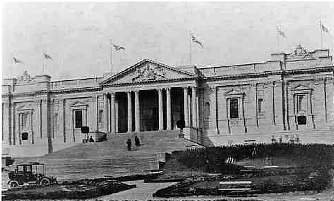
Figure 5.19. Comparison of St. Paul's, London, (above) and the British Pavilion, Edwin Lutyens. Lutyens was asked to copy the second story of St. Paul's for the Pavilion facade.
