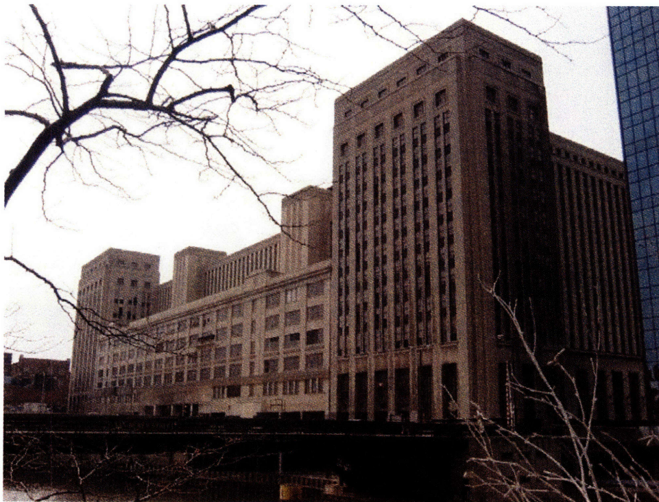
fig.29 A current view of the Old Post Office, from the downtown Loop.
