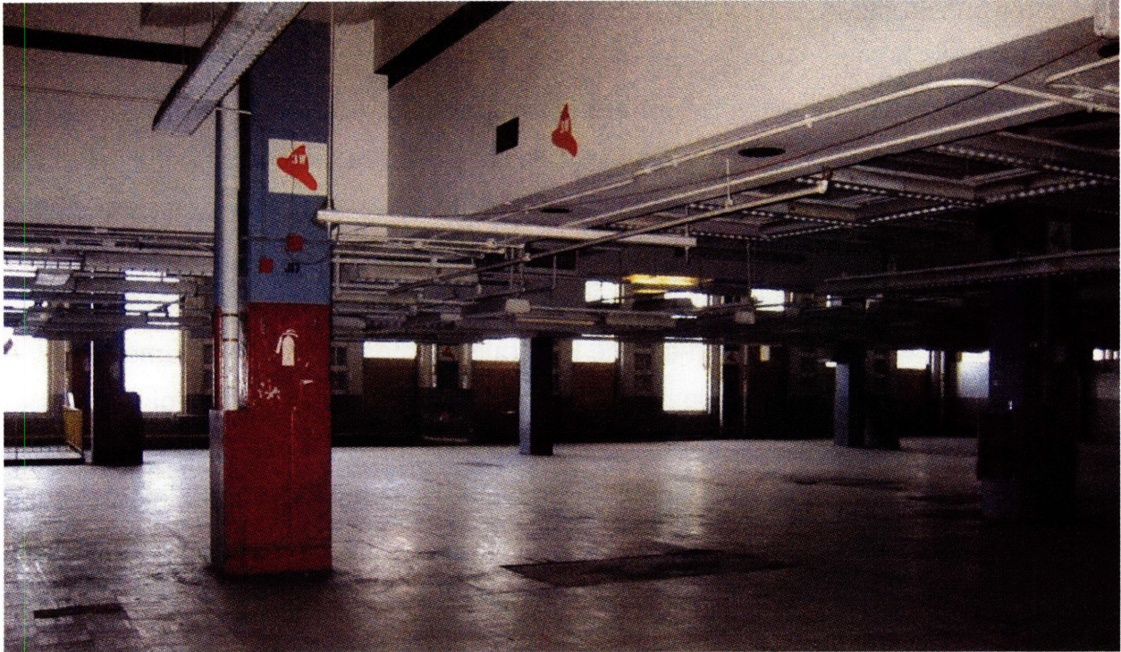
fig.34 Interior view of workspaces.
