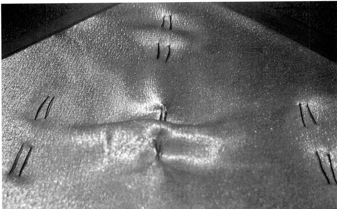
Figure 15 Structural wall clad in I/O textiles
