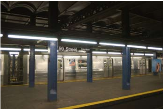
View across to abandoned center platform
