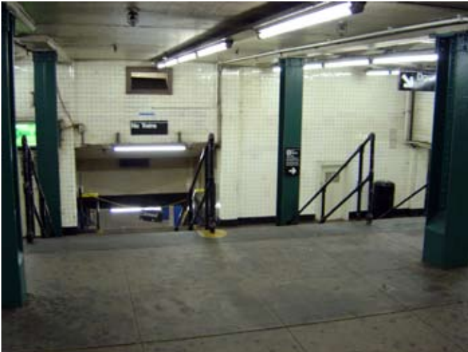
View from mezzanine/entry level to 'chained' stairs
