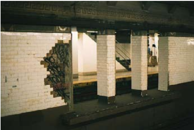
View from abandoned to active platform
