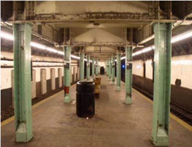
View looking down abandoned platform
